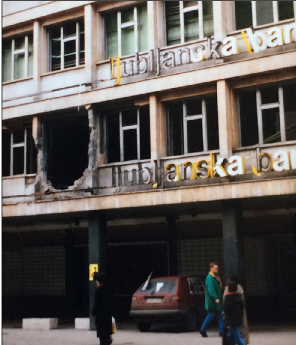
Typical random building damage in Sarajevo during the siege days. This is not the Salkic apartment building. Photo by Todd Bensman
