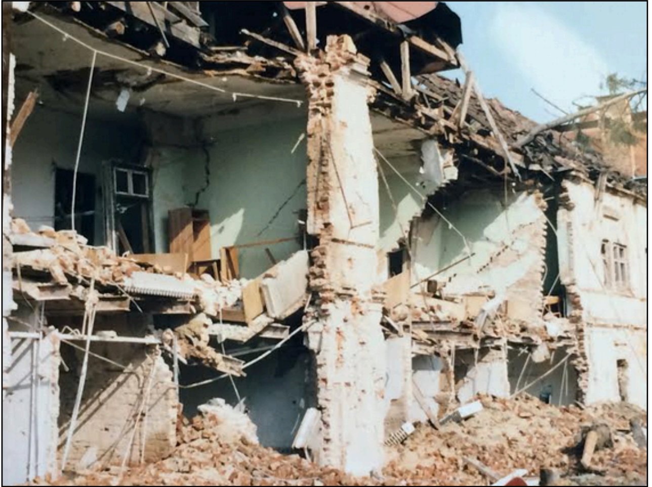
The destructive power of war in Bosnia shows in this ubiquitous home destruction in central Bosnia. Photo by Todd Bensman
